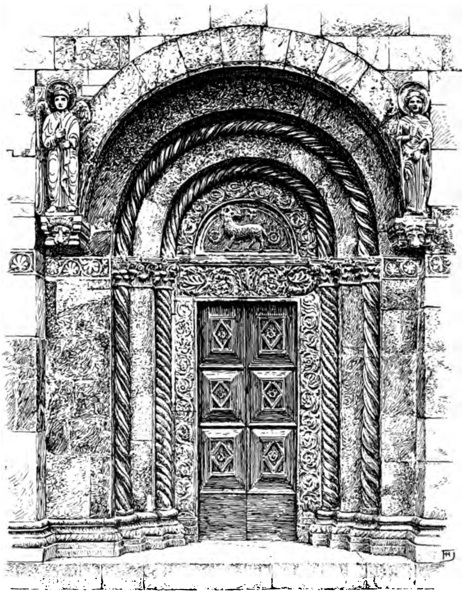
NORTH DOOR OF WESTERN FAÇADE, CATHEDRAL, ZARA
